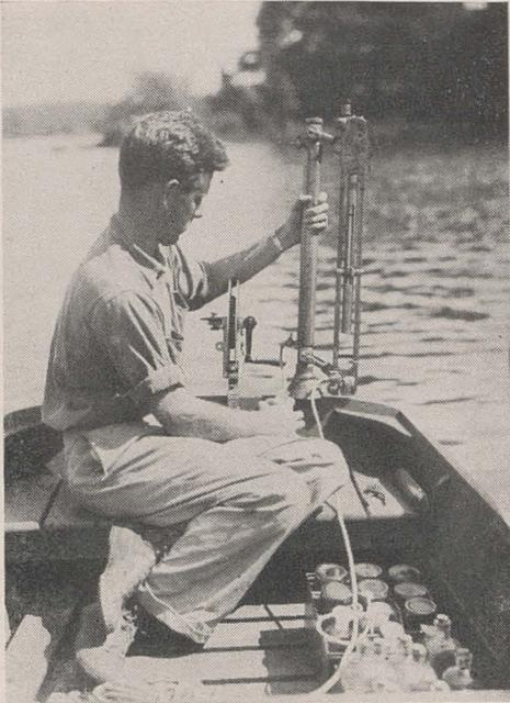
FIG. 10. One type of water sampling bottle and reversing thermometer.
