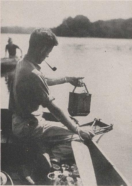
FIG. 12. The Ekman-Birge dredge is the apparatus used to obtain samples of organisms in soft mud bottoms.
