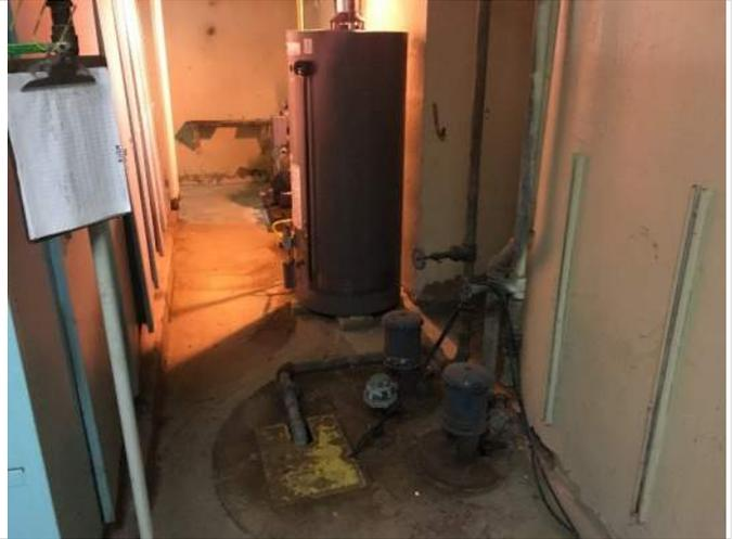
104. Control Building boiler room with natural gas hot water heater and sump.
