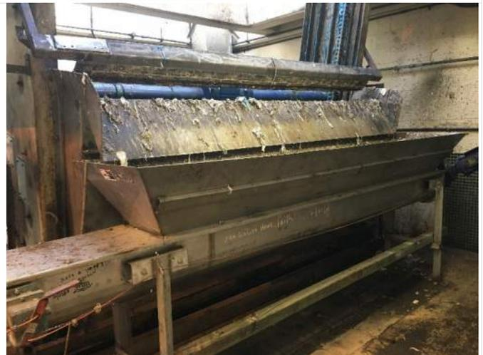
10. Screen Building screen hopper and debris processor.
