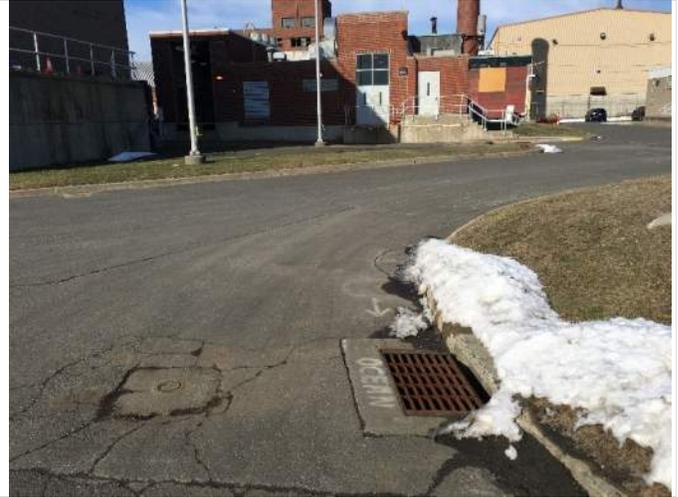
116. Typical Site catch basin connected to sanitary sewer system.
