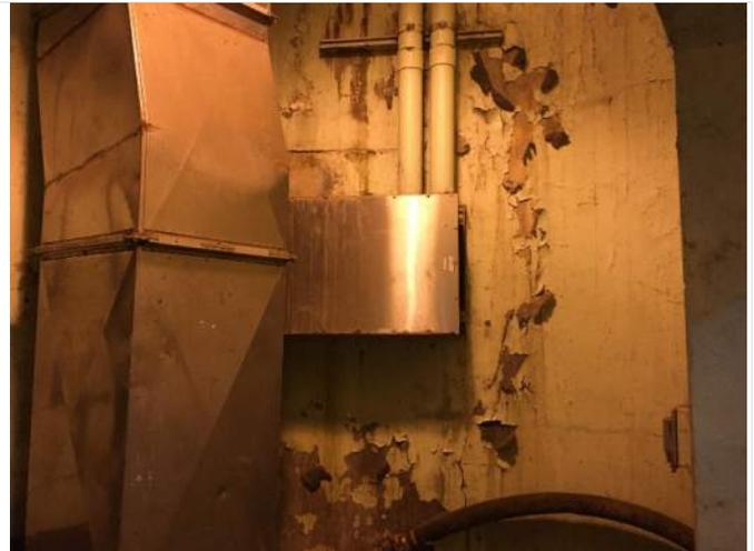
40. Pump Station lower level, peeling paint and suspect HBM.
