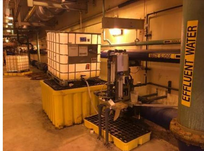
85. Pipe Gallery and typical effluent water supplemental chlorination system.
