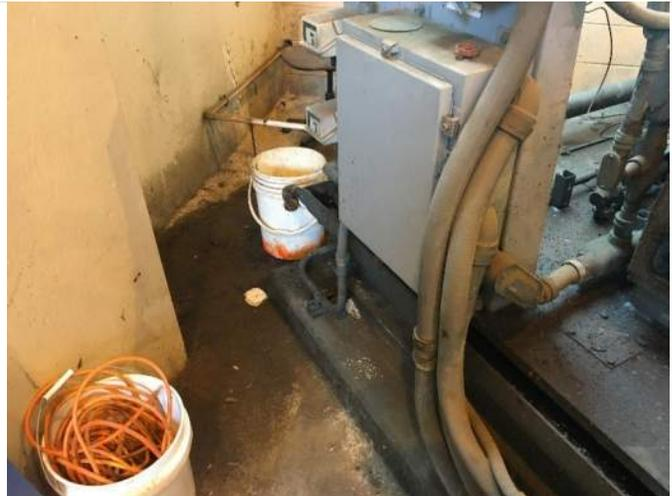
112. Control Building air circulation units with floor staining.
