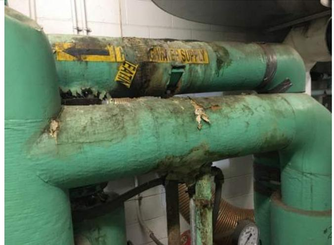
68. Degritter Building boiler room insulated piping and suspect HBM.
