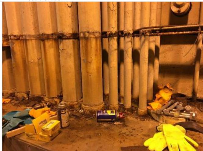
41. Degritter Building basement with debris and suspect HBM.
