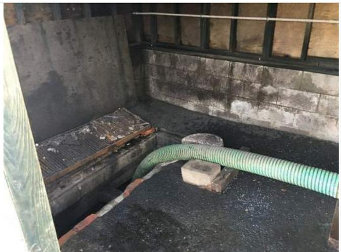
6. Inside the septic contractor dump station with drain to effluent flow.
