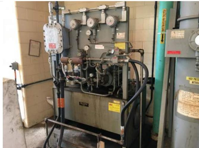
9. Screen Building main screen hydraulic system and hydraulic oil AST.
