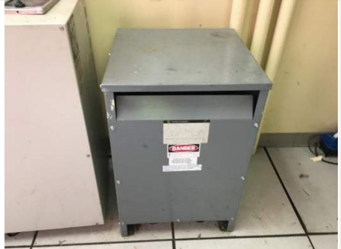
44. Pump Station control room and dry type transformer.
