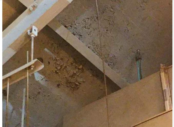
38. Pump Station ceiling, peeling paint, and suspect HBM.
