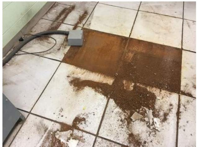
22. Screen Building control room with stained/damaged floor tiles/suspect HBM.
