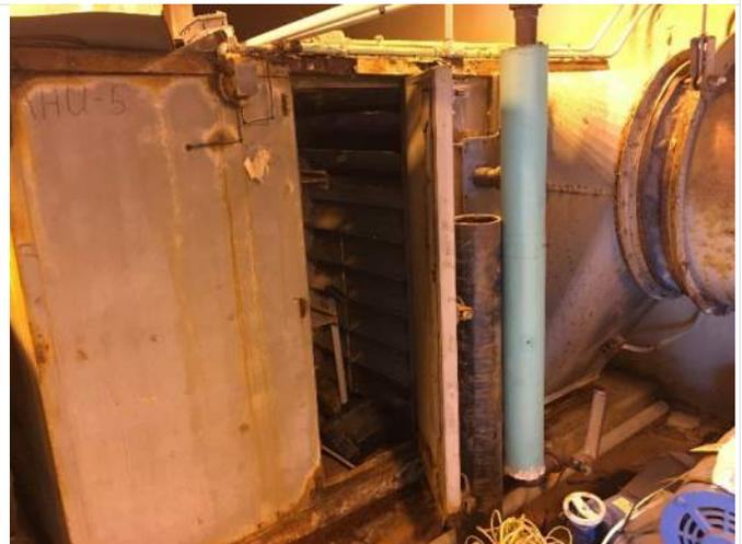
94. Pipe Gallery former air handling unit with suspect HBM..
