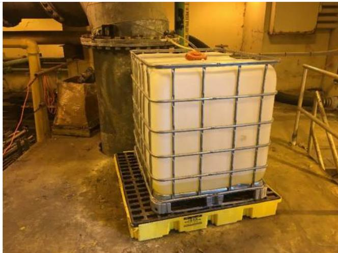
93. Pipe Gallery and typical effluent water supplemental chlorination system.
