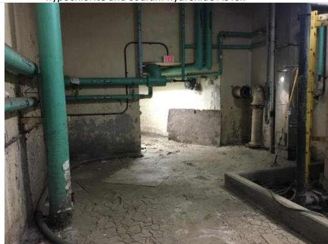
17. Screen Building basement and access tunnel to Pump Station. Substantial grit on the floor.
