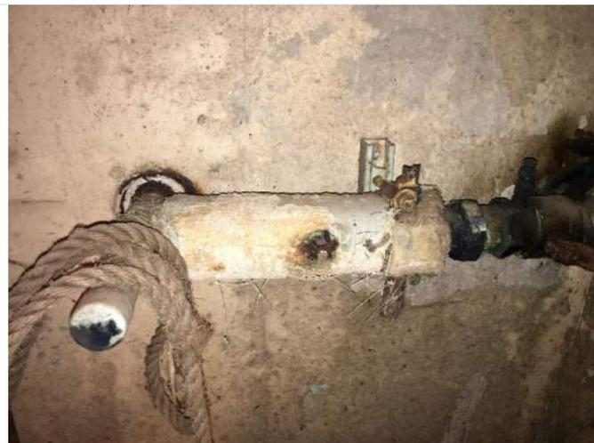
89. Pipe Gallery pipe insulation and suspect ACM.
