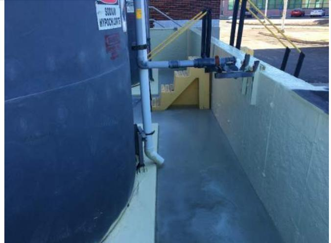
104. The facility's main sodium hypochlorite tanks and secondary containment.
