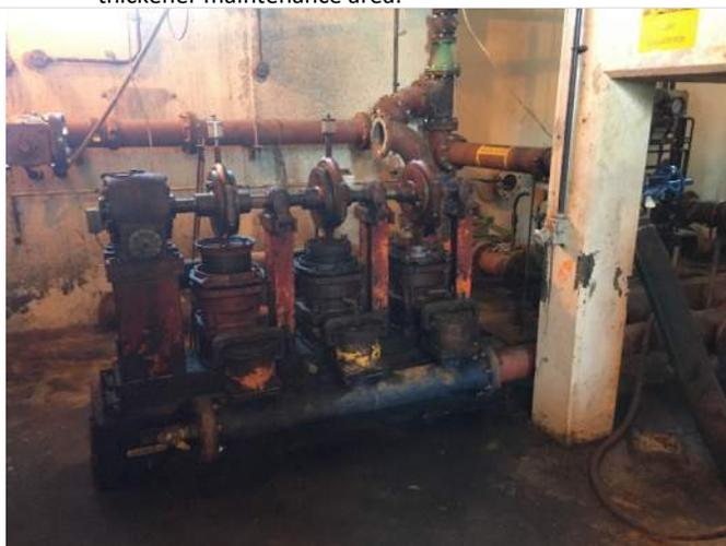
65. Out of service pump with floor staining inside the thickener maintenance area.
