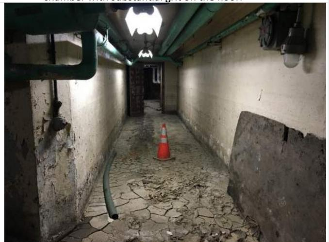
18. Screen Building access tunnel to Pump Station. Substantial grit on the floor.
