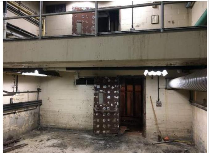
16. Screen Building basement and former grit collection chamber with substantial grit on the floor.
