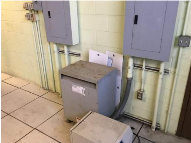
9. Typical control room, dry-type transformer and electrical panels.
